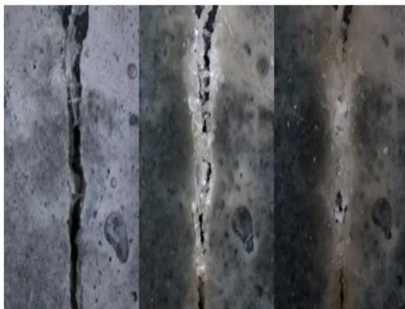
Crack Repair by Self-healing Concrete
